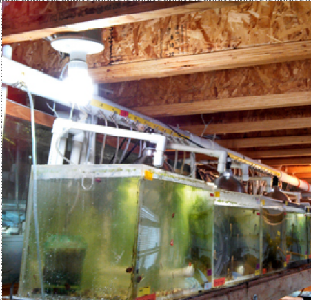
A central air system keeps the room organized and easy. 2 inch PVC should be used with air valves available at many online fish equipment suppliers.
