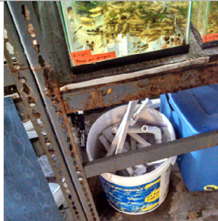
Metal racks will deteriorate in a humid fishroom. If ignored, entire legs can rust away, leaving the tanks holding one another up. You need to replace the racks before that happens!
